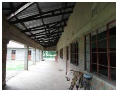
Illustration 4: Veranda and inner courtyard
